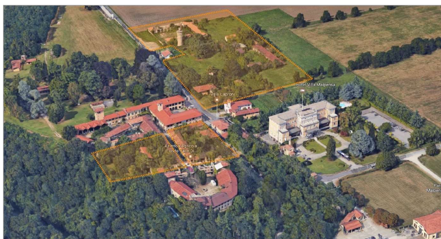
Aerial shot showing the areas involved in the project
